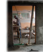
ICU in progress
